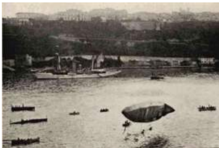
Phase D — before final collapse Accident, February 14, 1902
